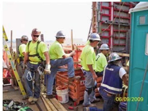
Figure 1. A 7th Floor Planning Meeting. Photos courtesy of Baker Concrete Construction.
